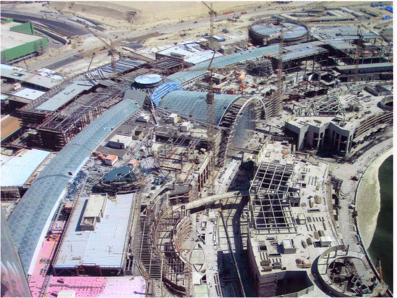
Dubai Festival City under construction
