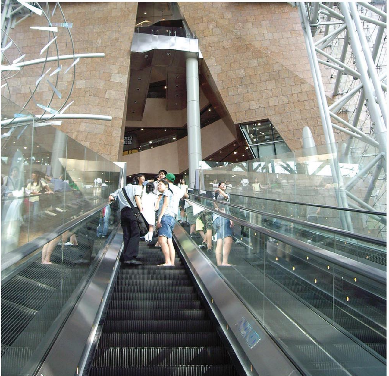
The Coopers smoke containment system protects the central atrium that spans several floors
