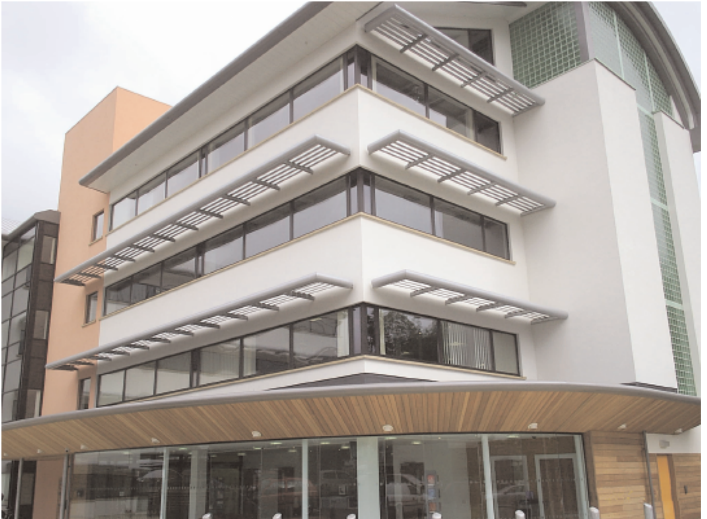
Brise Soleil fixed louvre sections fitted over the south and west facing windows of Swaythling Housing Association's new headquarters in Southampton.
